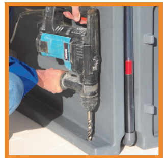
Drilling to secure a terminal to the floor
