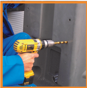
Drilling the cabinet to mount it on a wall or stand
